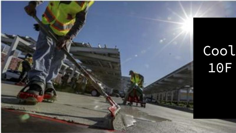
Cool pavement is 10F cooler than asphalt
